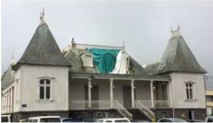
Figure 6 Tarpaulins Laid to Prevent Ingress of Rainwater
